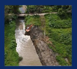
**Description-** Facilitated a project to collect the silt deposited and blocking the water flow of the river streams. The blocked river streams results in floods for the riverside communities and this project helped to mitigate that risk.
