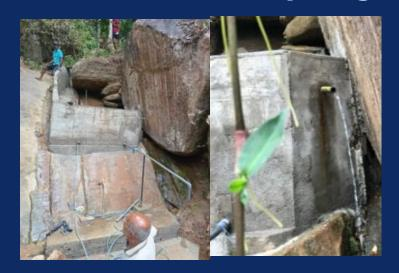
**Description-** Rehabilitate the spring well at Dippitiya. A water storage tank was build to collect the spring water flowing so as to allow the water to be used by the communities.
